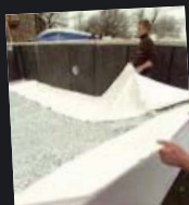
Fitting of the liner
