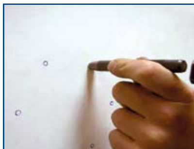
Cut through the liner with an 8 mm punch.
