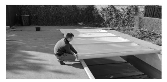
3. Determine the location of the cover to correctly locate the holes. Take into account the requirements of the overlay of 20 cm per side.
