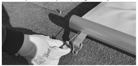
Drilling with the  $\emptyset$  10 mm drill, at a distance of 100 mm from the cover.
