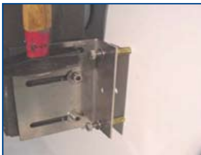
Slide plugs into drill holes and drive in with a bench hammer until bolt head touches bracket.
