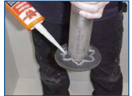
Apply sealant to gasket.
