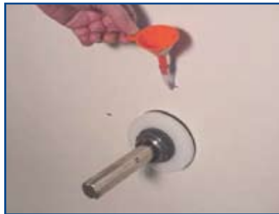
Fully insert funnel pouring hose into pouring channel.
