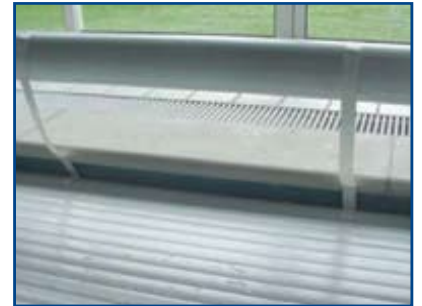
Fit the rest of the slats so the pool is completely covered (leave off any extras).
