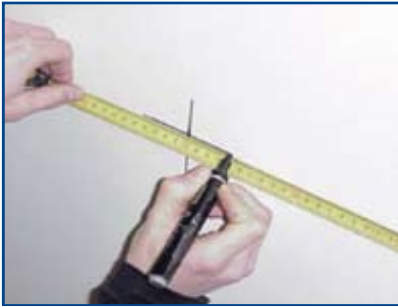
Mark the dimensions of the wall duct.
