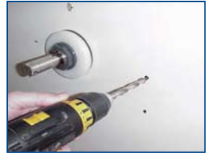
Drill Ø11 mm holes, at least 80 mm deep.
