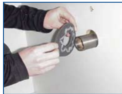
Fit gasket with sealant in motor well.
