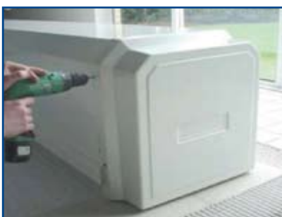
Fit the top cap and the side cover at the same time (drill to 4 mm and tap with M5).
