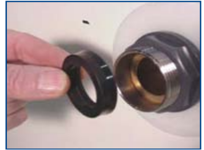
Place water seal on the well side with open side towards the pool.
