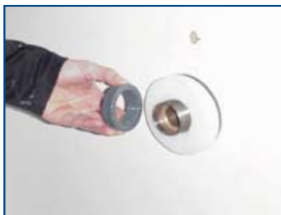
Fit check nut (hand tight).
