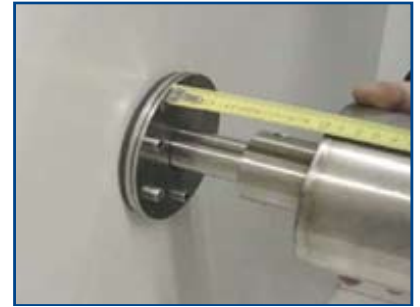
Determine length of spacer bush and cut to length.
