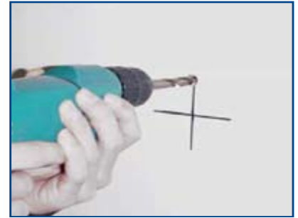
Drill first hole with \text{\O}11 mm drill. At least 80 mm deep.
