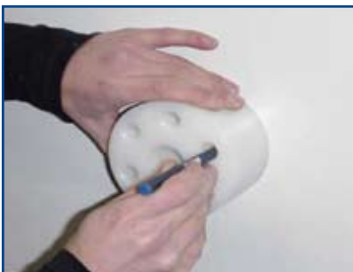
Insert plug, place bearing block and mark remaining holes.
